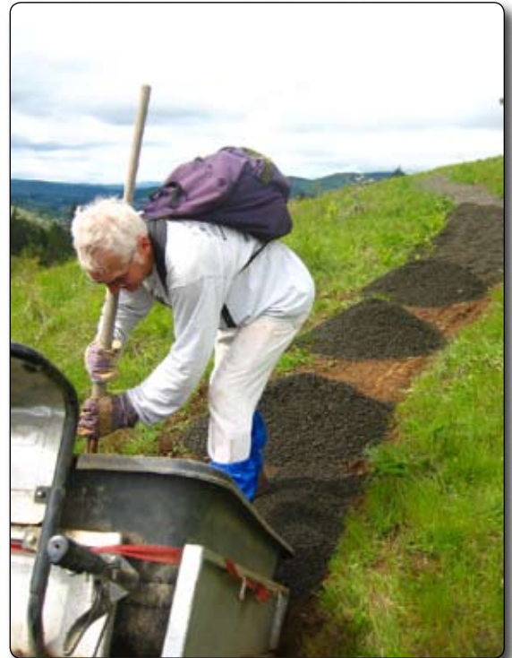
Trail building at Fitton Green Natural Area
