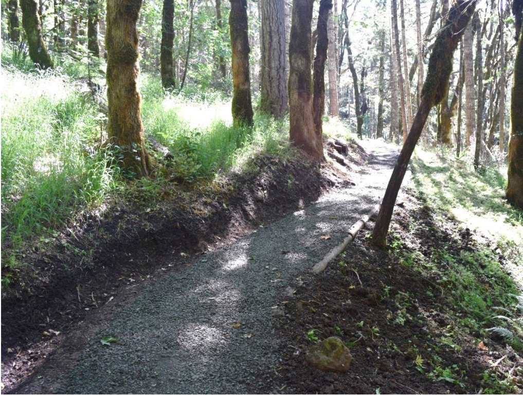
Figure 7. A view of the Mulkey Ridge trail. The tread is approximately three feet wide and composed of 3/4 inch minus gravel. Volunteers maintain the trail and interact with visitors.
